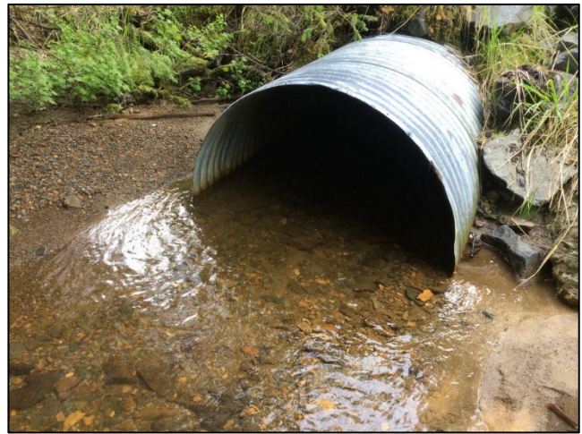
Figure 3.–Culvert at waypoint 101.
